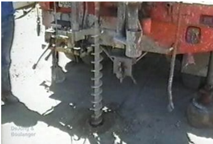
Solid flight augers may be used to install vertical groundwater and gas monitoring wells.
