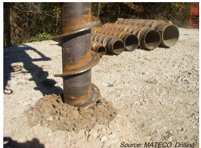
Hollow stem augers are preferred for undisturbed sample recovery and standard penetration testing, which are conducted from within the auger's interior space.
