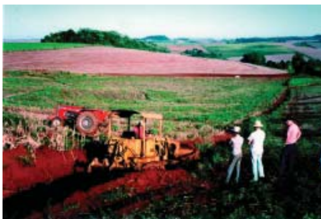
PLATE 45 Commencing the process of gully elimination
