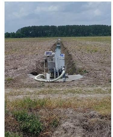
M Flashboard riser controls at the main line ditch exit point, shallow ditch system.
