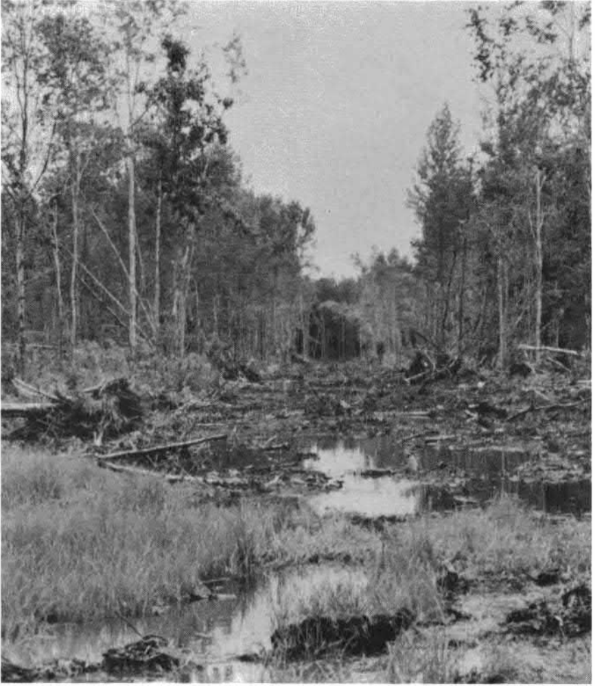
Figure 11. Right-of-way for a field ditch.
