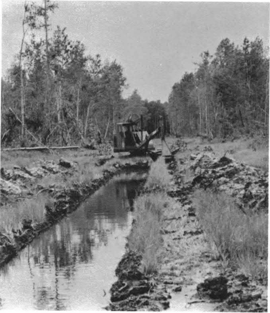
Figure 12. Field ditch being dug using a backhoe V-ditcher.
