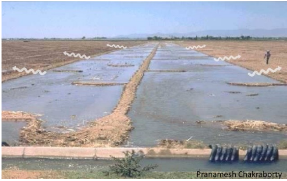
Figure 7.12.7 Surface irrigation infrastructure showing lines of seepage flow into adjacent crop lands. In arid regions seepage through irrigation canals like this can raise the water table in surrounding areas, impeding drainage, and causing salt build up via surface evaporation.
