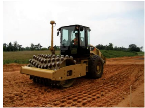
Figure 7.13.6 Sheepfoot roller compacting subgrade fill during road construction. Image source: pavementinteractive.org
